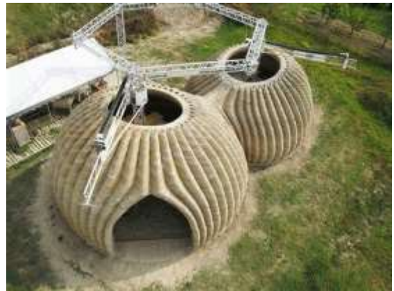
Figure (١5) showing the implementation of the TECLA house by three-dimensional printing
