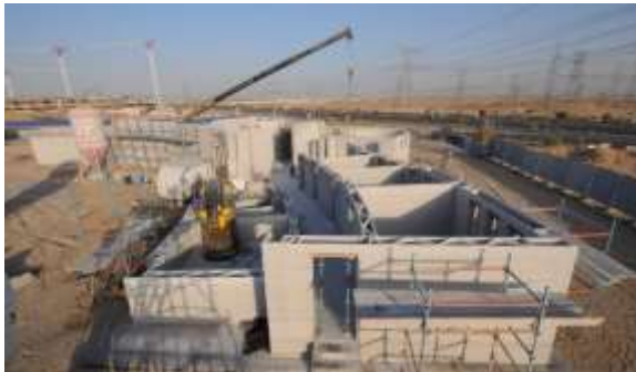
Figure (9) shows the implementation of the largest building in Dubai by three-dimensional printing technology
