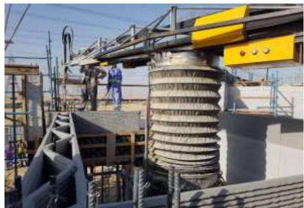
Figure (7) shows the method of building huge structures using three-dimensional printing
