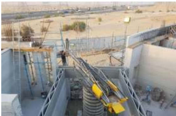
Figure (10) shows the implementation of the largest building in Dubai by three-dimensional printing technology
