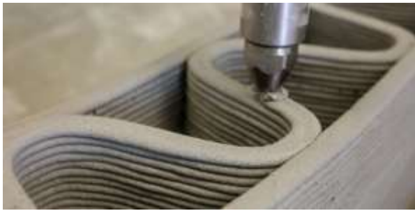
Figure (13) shows the method of extrusion in three-dimensional printing
