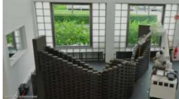
Figure (3) shows the working robot and a robot that performs work in construction sites where it can stack bricks to complete construction operations
