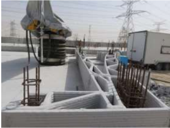
Figure (8) shows the method of building huge structures using three-dimensional printing
