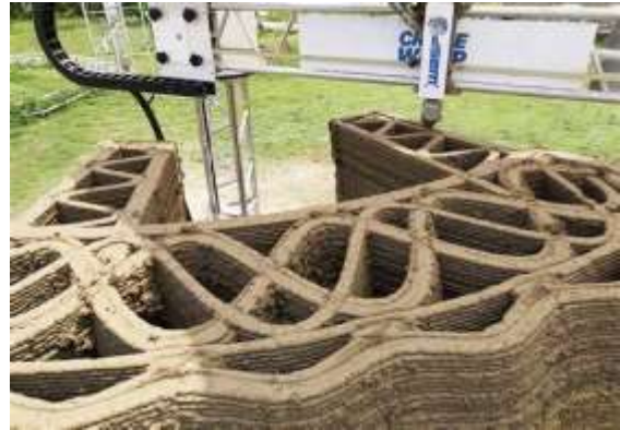
Figure (١٤) showing the implementation of the TECLA house by three-dimensional printing
