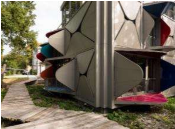
Figure“17”: Structure System of movable panels are composed of rigid steel cantilever beams covered with aluminum sheets
