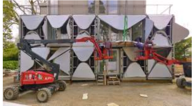
Figure“17”: Structure System of movable panels are composed of rigid steel cantilever beams covered with aluminum sheets
