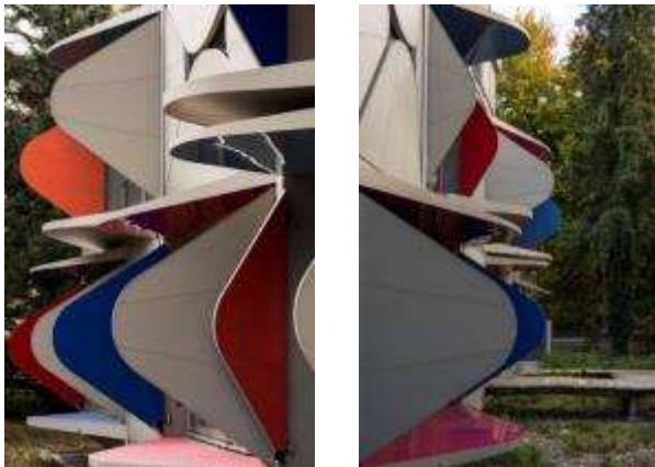
Figure“16”: Hinged movement panels (shutters) on the facade (open-close) as needed .
