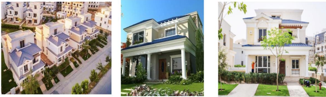
Figure (6): Description of the villa, Fifth Square, Source: https://mountainviewegypt.com/projects/2-mountain-view-ii
